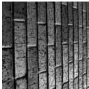
(a1) Brick wall
